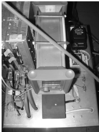
Fig. 3: Engine control unit (left) and charge amplifier (center) in opened device box
